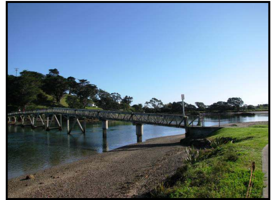
Pictured above - Pataua foot bridge
